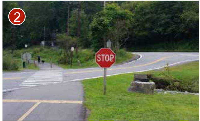
2 A tighter turning radius at the Deckers Creek Boulevard / Powell intersection would improve safety for trail users crossing here
