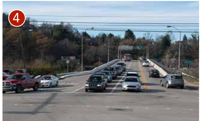
4 With the indefinite closure of River Road, only one lane of traffic feeds the Westover Bridge (southbound), where three traffic lanes provide no space for bicyclists
