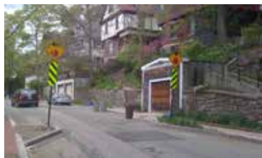
Chokers create pinch-points that reduce speeds mid-block.
