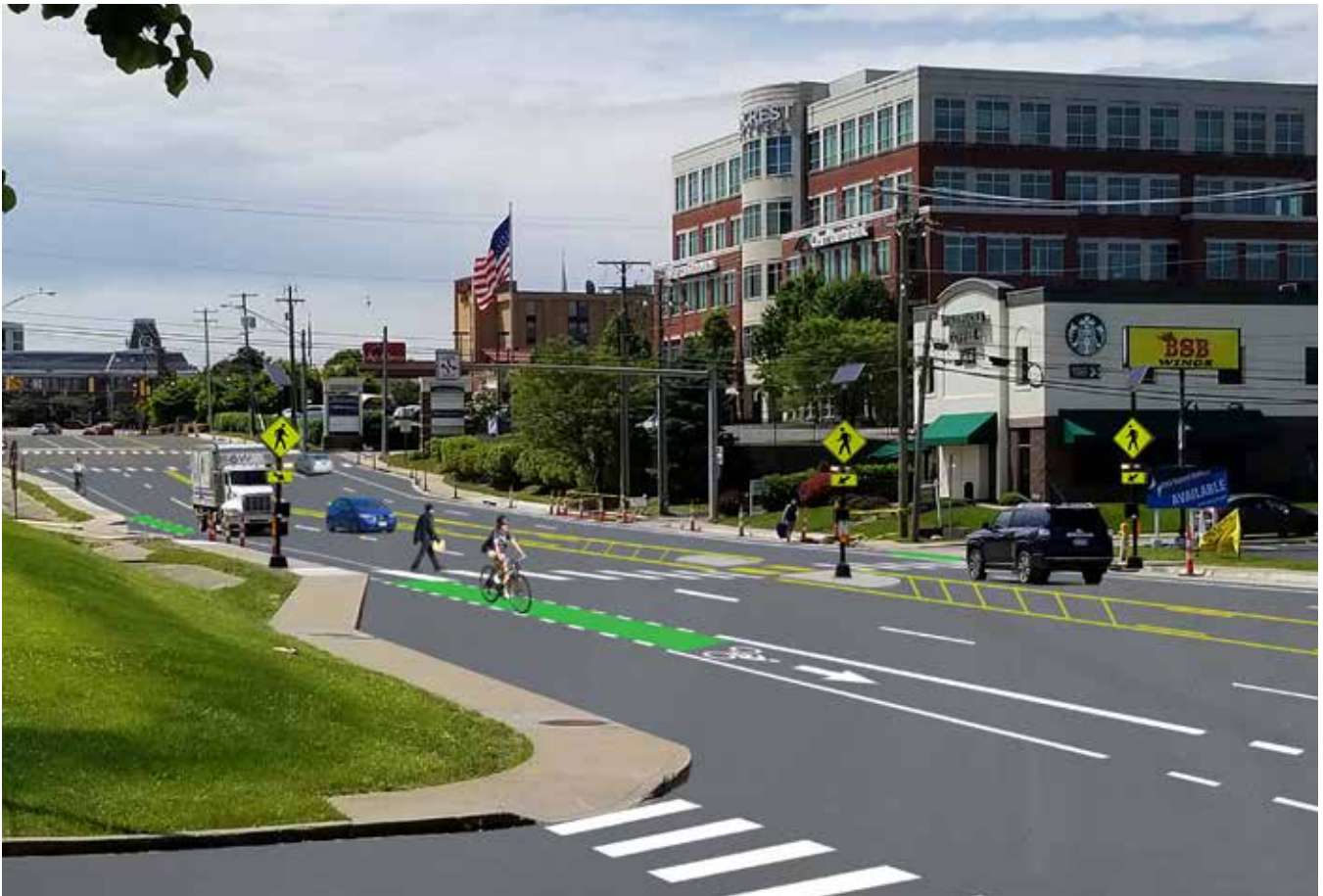
Narrower travel lanes on Route 705 provides space for striped bike lanes and the turn median accommodates a raised median island to improve the level of safety—along with the RRFB—for the recommended crosswalk
