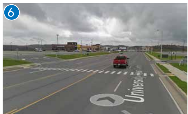
6 Though not a pedestrian gap per se, crossing 5-lane-wide University Town Center Drive on foot remains a challenge without additional safety measures other than a striped crosswalk
