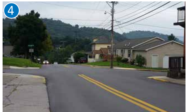
4 Lack of crosswalks at the intersection of Richwood Ave and Putnam Street create a gap at an important bus stop location
