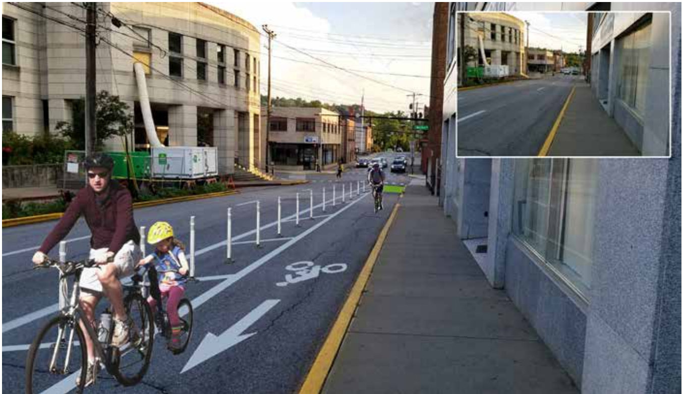
A buffered bike lane along Spruce Street benefits pedestrian traffic by providing a wide spatial buffer for the adjacent sidewalk
