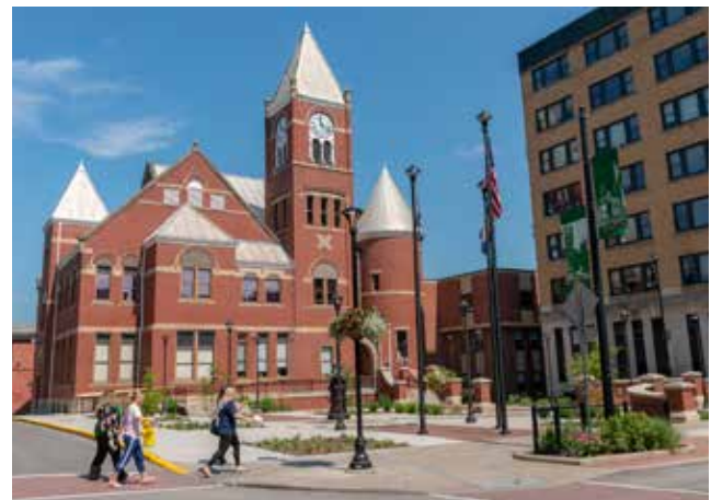
Monongalia County Courthouse building and plaza
