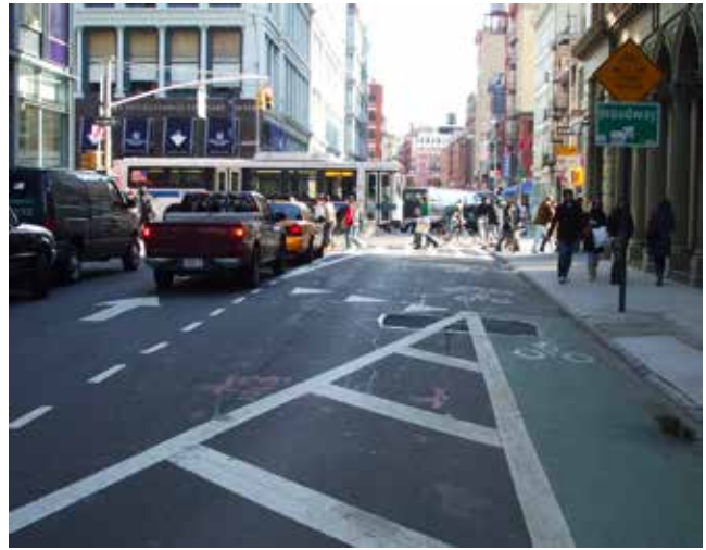
Image of combined bike and turn lane in New York City
