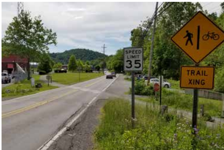
Proposed recommendations include a revised crossing geometry for the trail, along with a RRFB for enhanced safety
