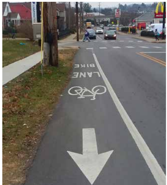
Climbing Bicycle Lane on University Avenue
