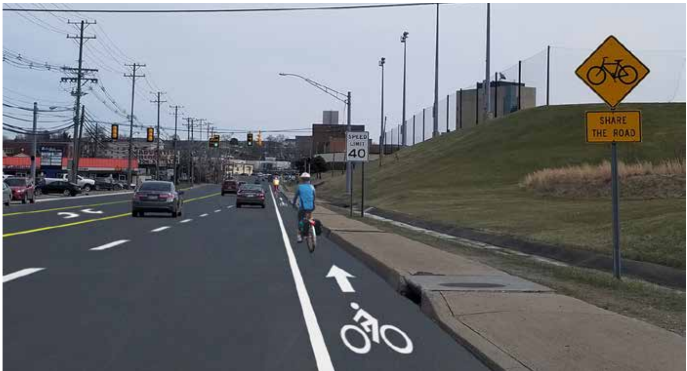
By narrowing Route 705 travel lanes to 11' in width, space becomes available for striped bike lanes in each direction
