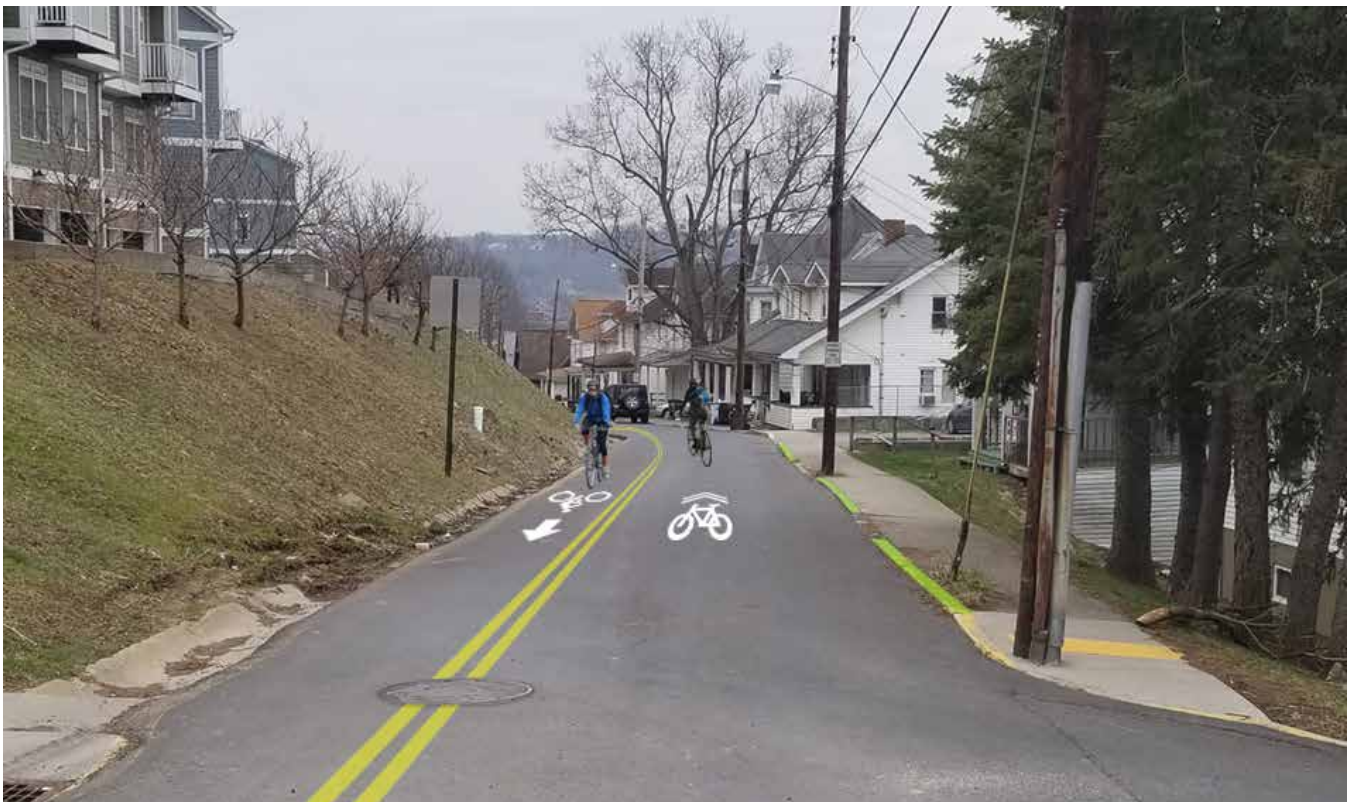
Currently, the City of Morgantown is moving forward with the implementation of a contra-flow bicycle climbing lane on Jones Avenue
