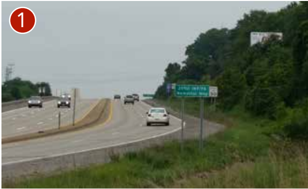
1 High traffic volumes and speeds on 201st Inf / FA Memorial Way likely necessitates a facility separated from the roadway on the north/east side for pedestrian and bike access
