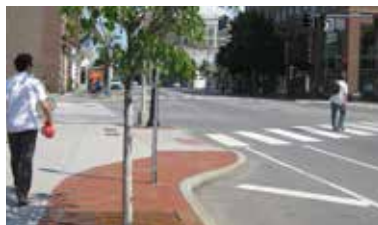
Curb extensions reduce turn radii, turning speed, and reduce pedestrian crossing distance.
