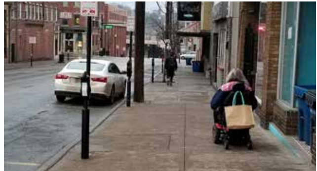
Existing sidewalk downtown
