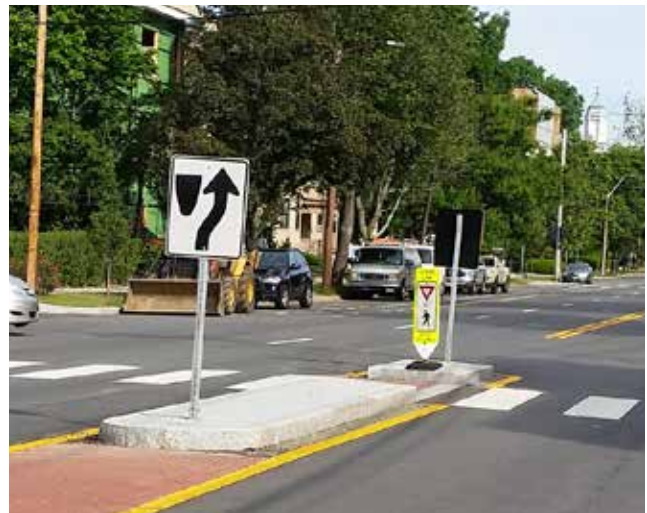
Median refuge island
