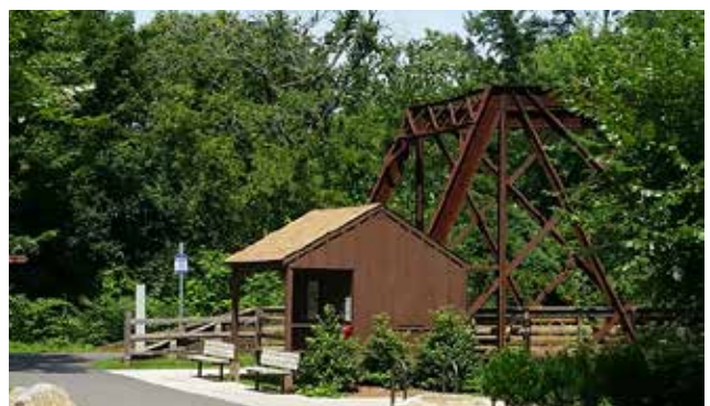
Example trail access point
