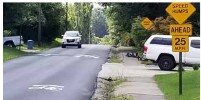
Bike Boulevard on Jr Avenue in Morgantown
