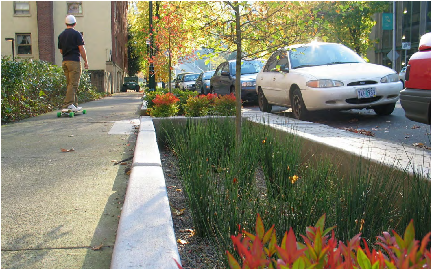
Stormwater infiltration areas (green streets infrastructure).
