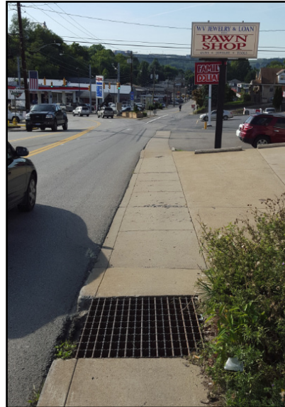
Sidewalk on Holland Ave near the Westover Triangle
