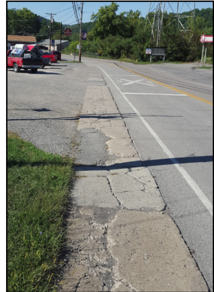
Sidewalk connecting Westover and Granville
