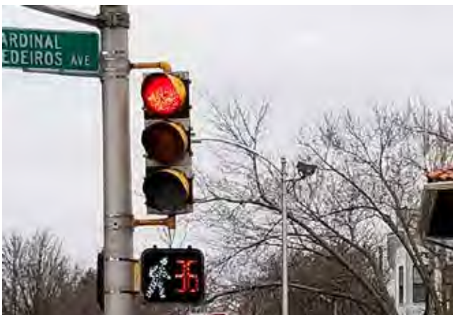
Pedestrian Countdown Signal with Lead Pedestrian Interval
