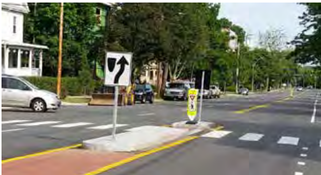
Median Refuge Island
