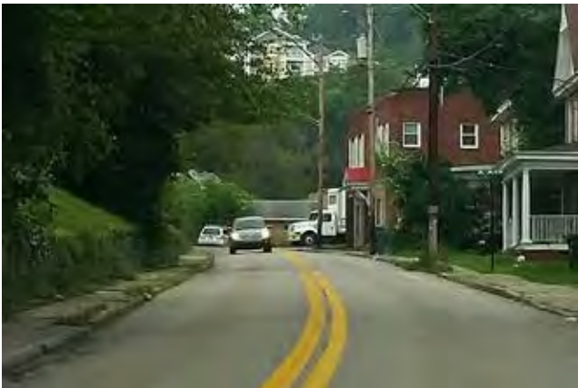
Sidewalks in need of repair on Willey St in Morgantown
