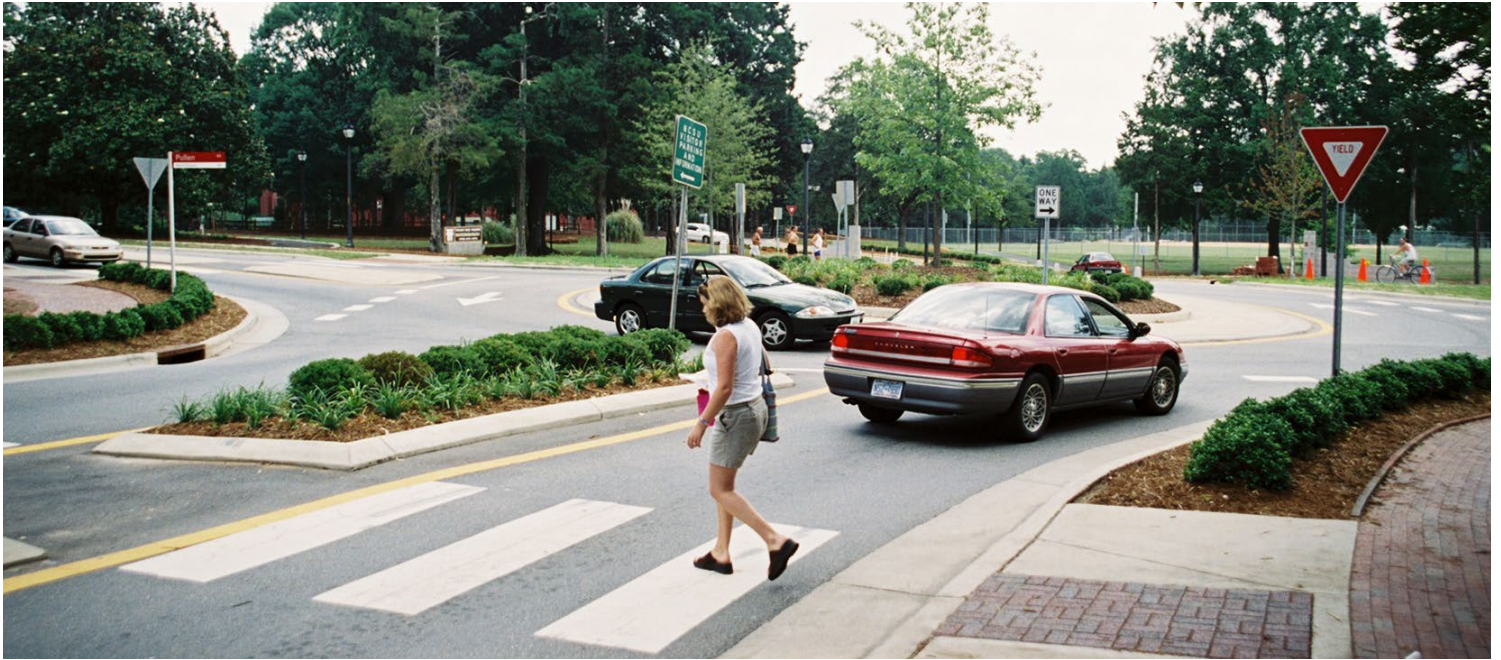
Roundabouts are one example of an intersection safety improvement.
