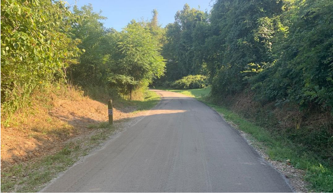
Decker's Creek Rail-Trail.
