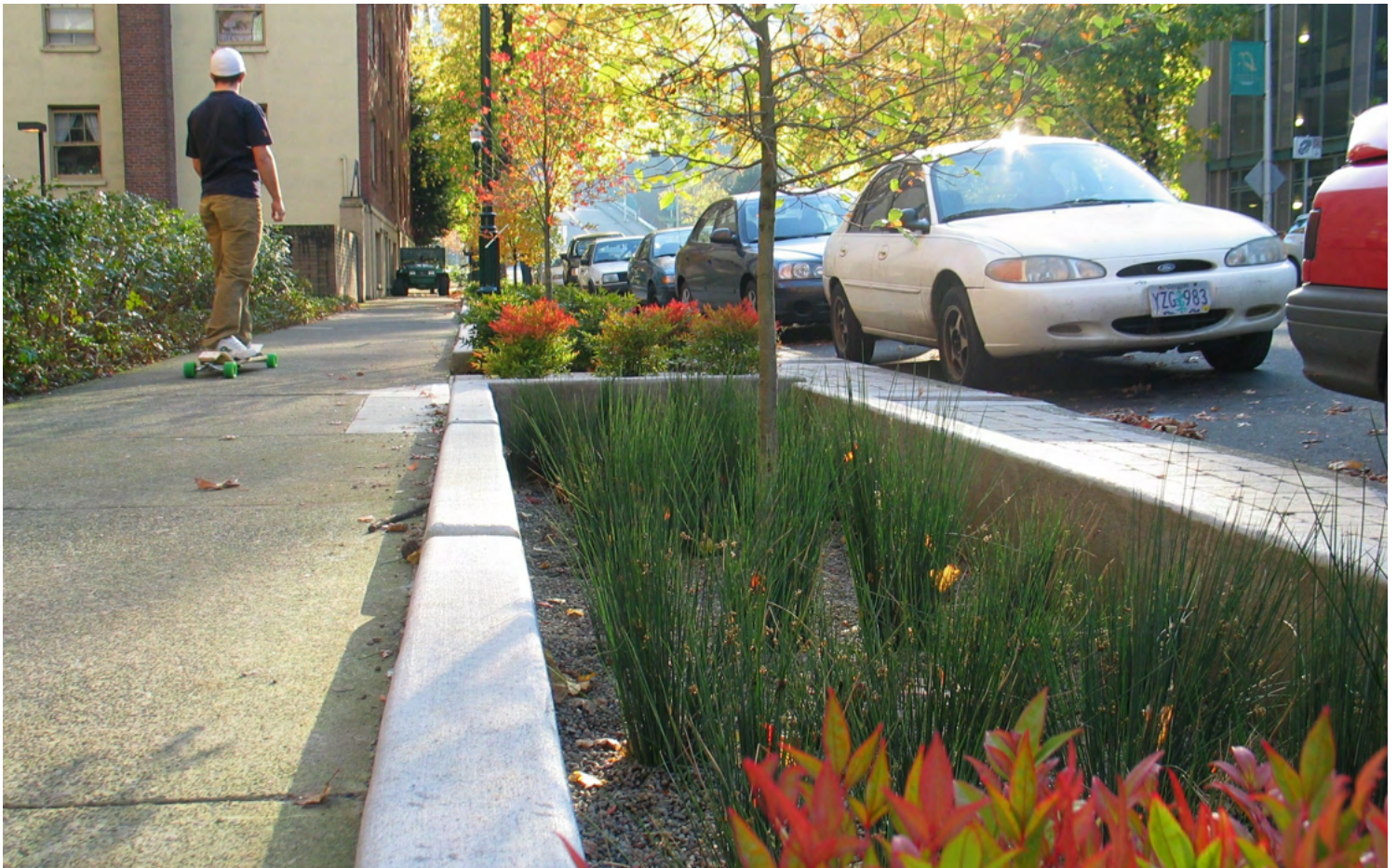
Stormwater infiltration areas (green streets infrastructure).
