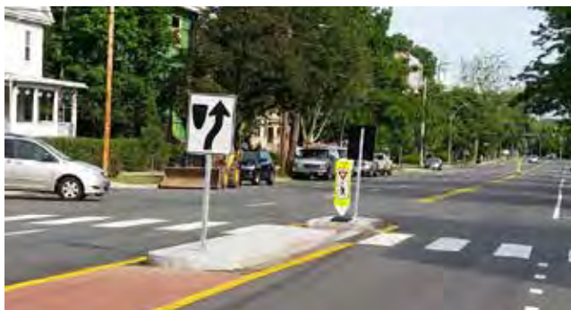
Median Refuge Island
