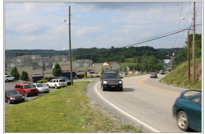
Figure 3. Three-Lane Section with Climbing Lane
